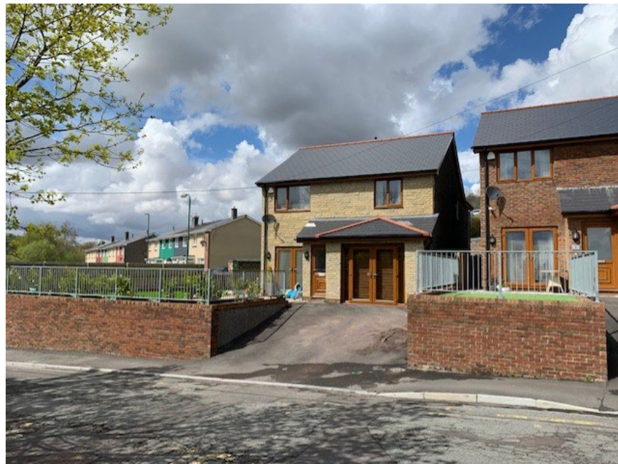
Photograph 6: showing how side boundaries to the front of building lines have been demarcated by rendered walls and galvanised railings
