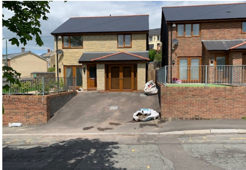
Photograph 4: showing front elevation of 1 Rhes yr Ysgol finished in reconstituted stone.
