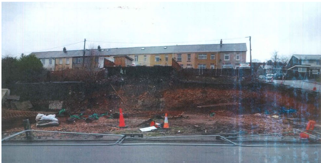
Photograph 12: showing site excavations prior to construction works commencing
