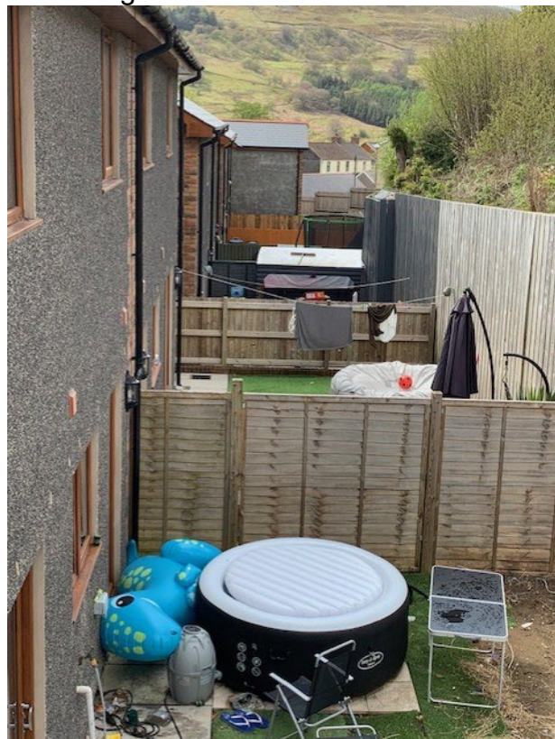
Photograph 8: showing the timber fence side boundaries between properties and a section of the new retaining wall constructed along part of the northern boundary with elevated garden areas relating to Gwent Terrace above.
