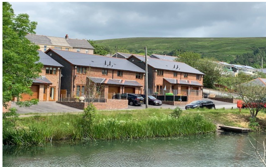
Photograph 3; showing front elevations of 3-7 Rhos yr Ysgol finished in brickwork
